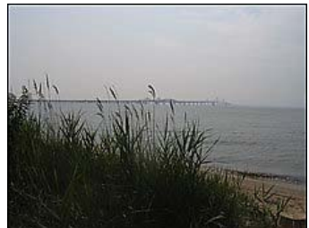
A view of the Chesapeake Bay Bridge from Kent Island, Md. (Zofia Smardz - By Zofia Smardz)
